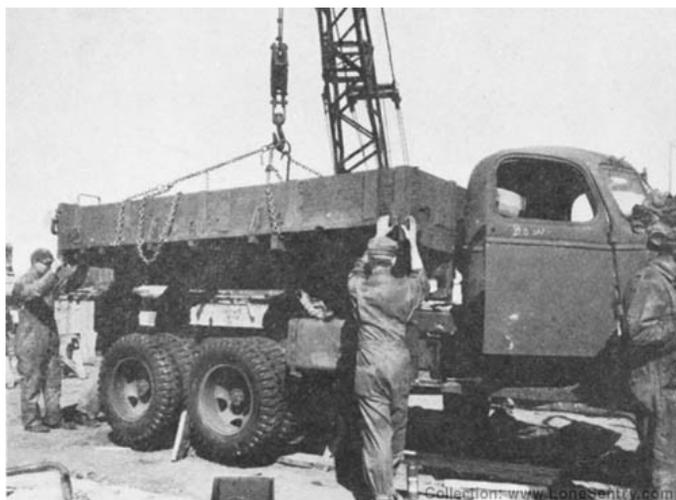
A crew of ten to twelve men would assemble the entire vehicle in as little as an hour, test drive it, and then turn it over to a unit. In the Mediterranean Theater of operations alone, they assembled 126,669 vehicles.
